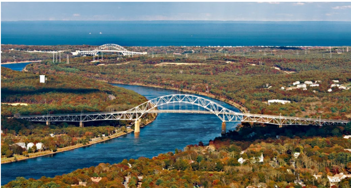
Figure ES-6 – Looking Northeast at the Bourne and Sagamore Highway Bridges
